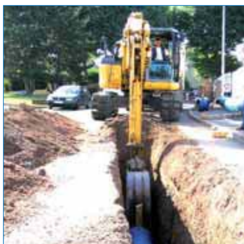
Locking a STANDARD Vi anchoring system with the bucket of a digger
