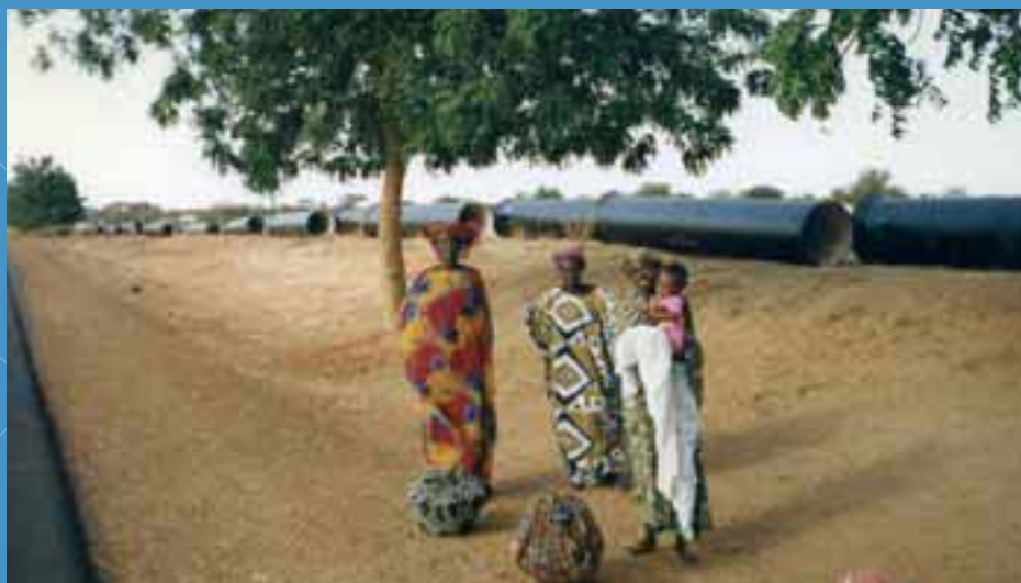
Delivery of ductile iron pipes for the supply of drinking water to Dakar (Senegal).
