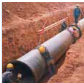
Laying of a water supply pipe
