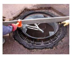
7 Check that the frame openings have been completely filled.
