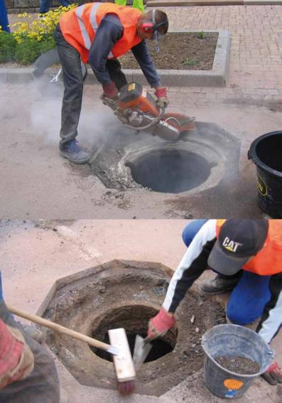
1 Check the diameter of the manhole opening or groove that the frame is to be fitted on.
