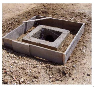
Check the condition of the manhole opening or groove, removing any debris, loose particles or dirt (oil, grease, etc.).
